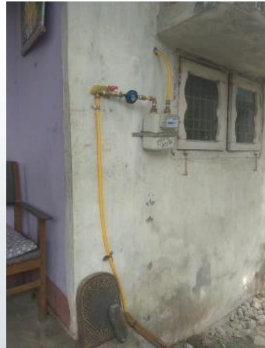
Metering system used in households
