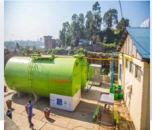
Continuously Stirred Tank Reactor (CSTR)
